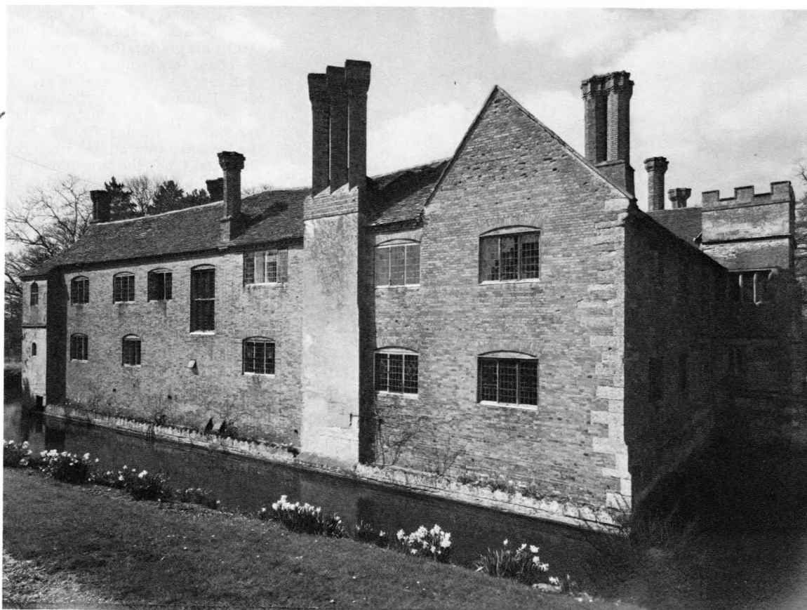
4—THE EARLY-18th-CENTURY SOUTH RANGE. "If removed from its moat, it could be taken for a substantial Warwickshire Georgian farmhouse"
